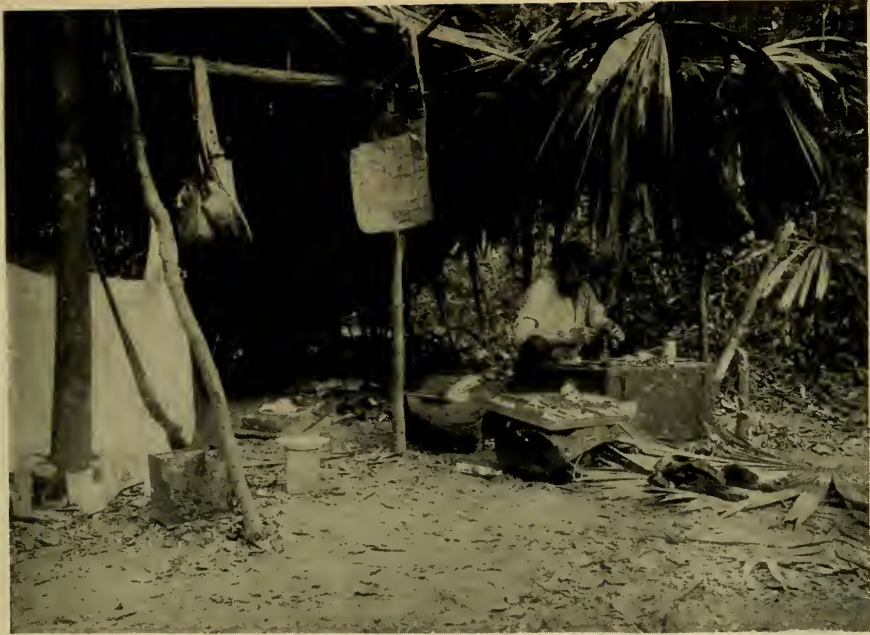
FIG. 1.—Camp on Cerro Azul. A palm-thatched roof affords shelter from the hardest rain.
